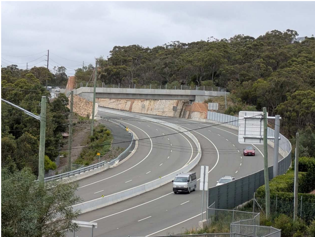
Fauna bridge on Mona Vale Road East. Ingleside Chase Reserve is on left. Photo David Palmer
